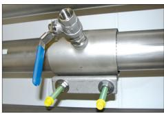
If there is no measuring site with 1/2" ball valve present on existing pipes, it can be set up quickly and cost-effectively by means of spot drilling collars. The spot drilling collar is imposed onto the pipe and tightened via thread rods. The enveloping rubber gasket is pressure-tight up to 11 bar. By means of the drilling jig, it is possible to drill the spot drilling collar through the 1/2" ball valve into the existing pipe.
