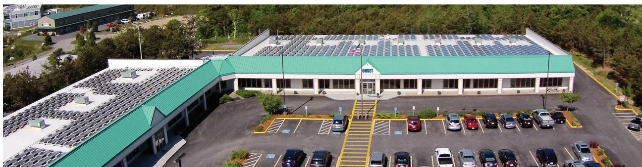
Onset headquarters, Cape Cod, MA
