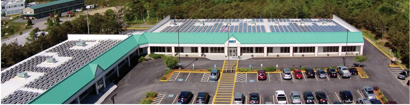
Onset headquarters, Cape Cod, MA
