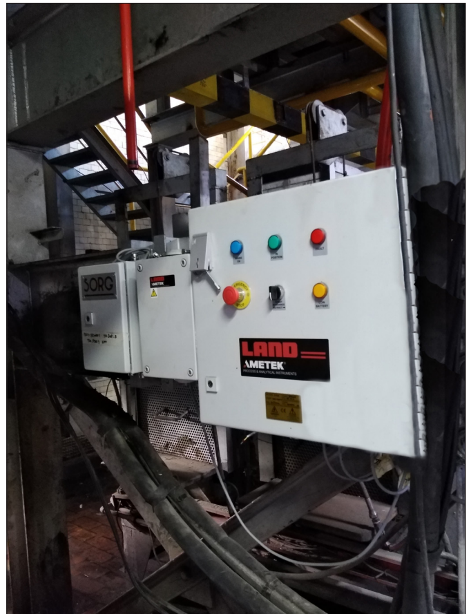
NIR-B-656-Glass System Installation
